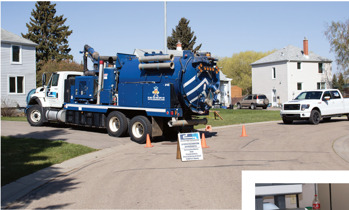
Left: When Canessco arrives on a job with the Vac-Con rigs, workers place cones and signs around the work site to protect technicians and passers-by.
